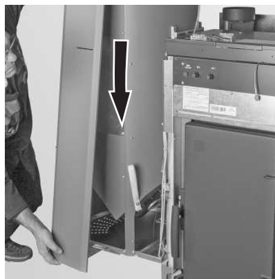
Fig. 66 Push down the cover and remove (bayonet lock)
