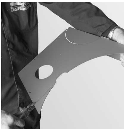
Fig. 74 Pinch off the corner of the cladding at top left
