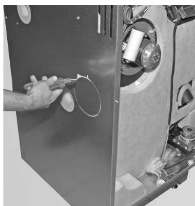
Fig. 29 Punch out the cut-out
