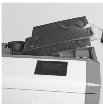
Fig. 63 Remove the insulation
