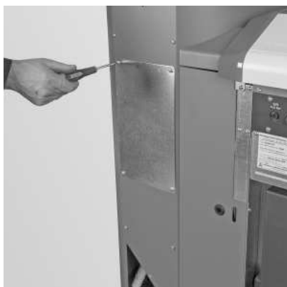
Fig. 67 Remove the screws and take off the inspection cover
