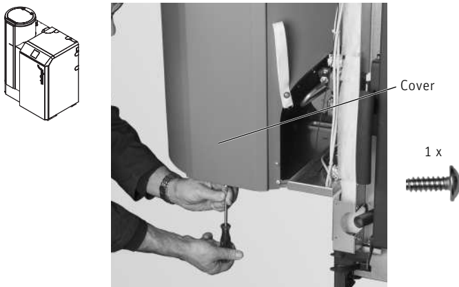
Fig. 53 Attach the cover and secure with 1 self-tapping screw
