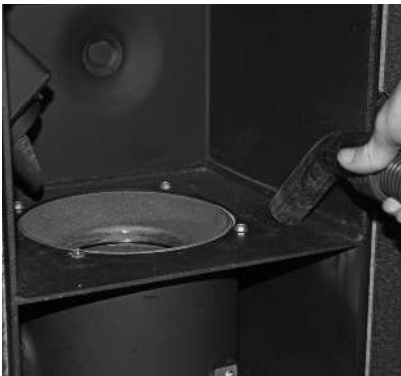
Fig. 39 Remove combustion residue from the combustion chamber
