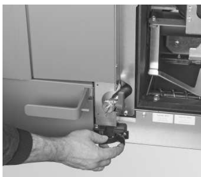
Fig. 32 Open the bracket fastener
