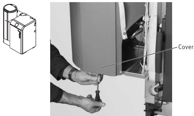
Fig. 45 Dismount the cover, removing 1 screw
