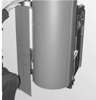
Fig. 64 Remove the adhesive tape from the water tank and hook on the cladding
