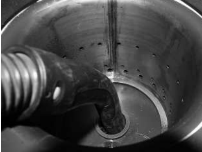
Fig. 48 Vacuum out the primary air tube in the centre of the burner bowl
