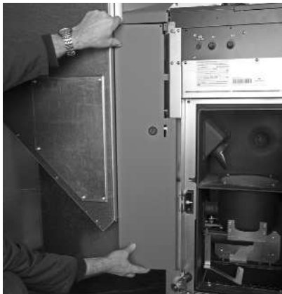
Fig. 78 Insert the front cladding
