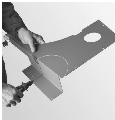
Fig. 75 Punch out the cut-out only if the flue connection is at the top
