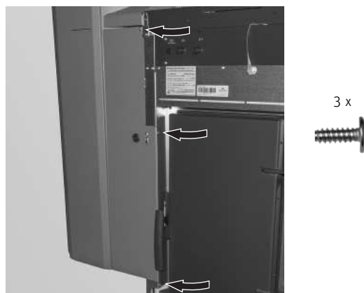
Fig. 69 Secure the front cladding with screws
