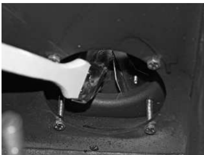
Fig. 56 Clean and vacuum the induced draught fan wheel
