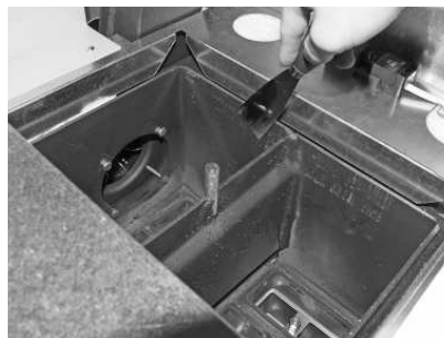
Fig. 57 Clean the heat exchangers
